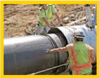
Using chains and pressure from the excavator, the two pieces of pipe are 'snapped' together. The process is repeated until connected sections of Snap-Tite® are pushed through the entire length of the culvert.
