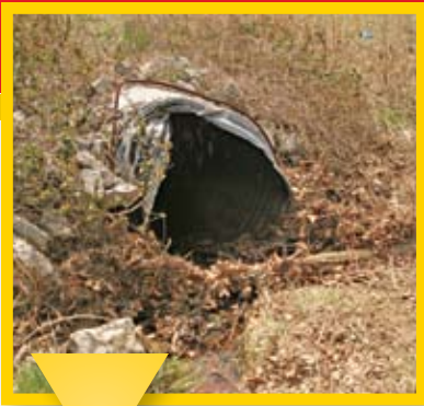
A typical deteriorated culvert close to failure, potentially leading to road collapse and danger to the motoring public.
