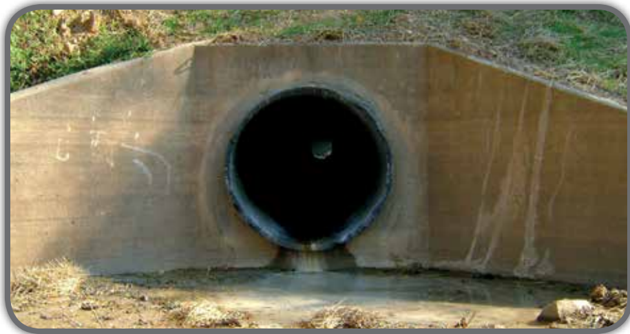
After rehabilitation with Snap-Tite®
