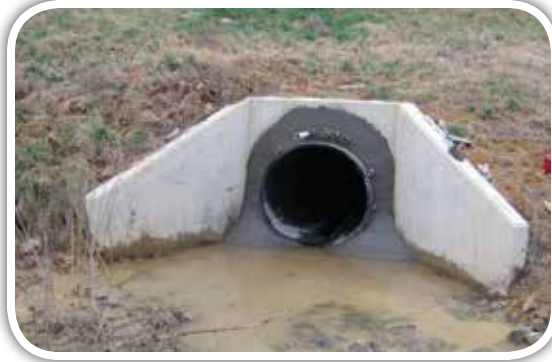
The above picture shows sliplining through a wing wall. An end seal with fill pipes is under construction.
