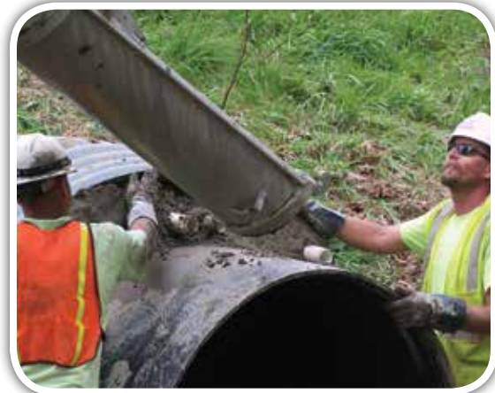
Cast in place headwall
