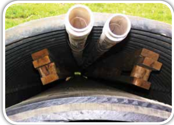
Pieces of wood are used to maintain grade and alignment
