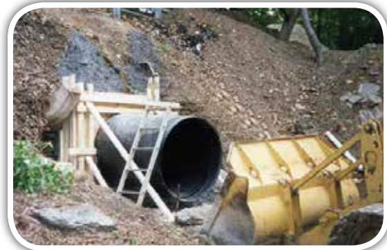
Cast in place headwall
