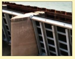
580 megawatt combined cycle power plant needed a non-metallic trashrack with galvanized steel framing to fit it's existing intake.
