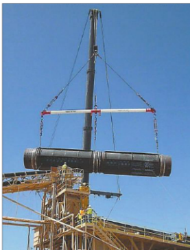
Hydro Watt's construction team lifts a trommel they built.
