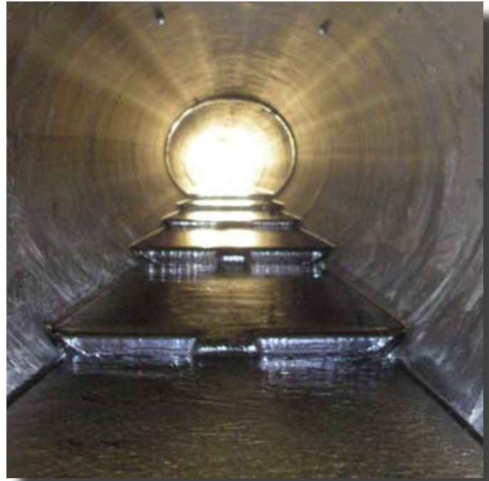
Ponding effect created by baffle/weir design during low flow.
